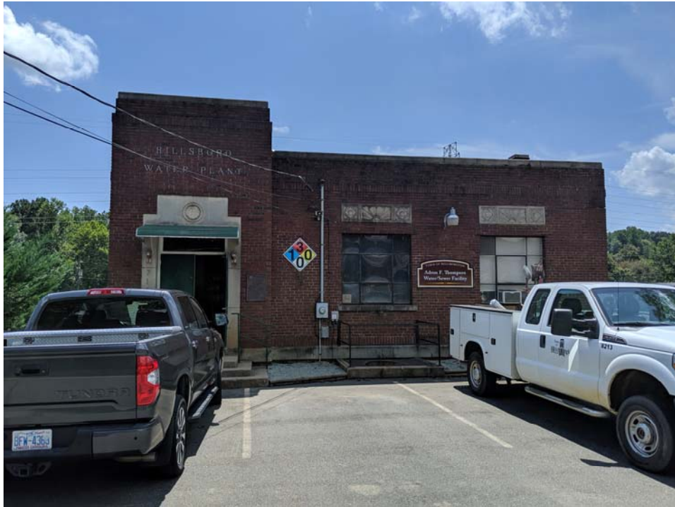
715 Dimmocks Mill Road Water Plant A Side
