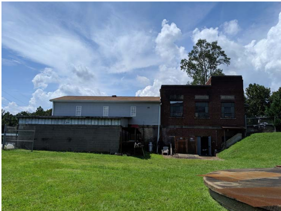
715 Dimmocks Mill Road Water Plant B Side
