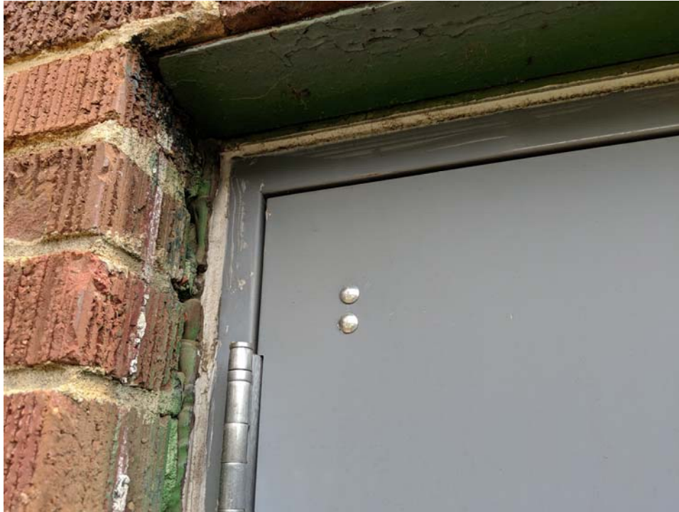
Door caulk on original brick structure.
