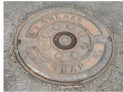
Water from sinks at this coffee shop (left photo) drains into a grease trap (bottom left) to prevent fats, oils and grease from entering the sewer system. Above is the access to an exterior grease trap at a restaurant.
