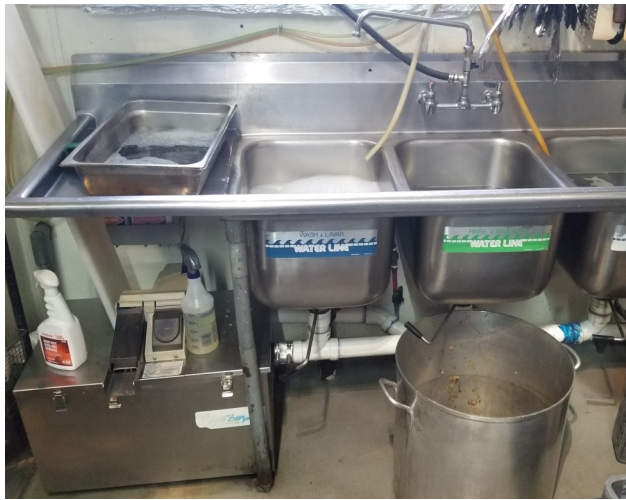
Water from sinks at this coffee shop (left photo) drains into a grease trap (bottom left) to prevent fats, oils and grease from entering the sewer system. Above is the access to an exterior grease trap at a restaurant.
